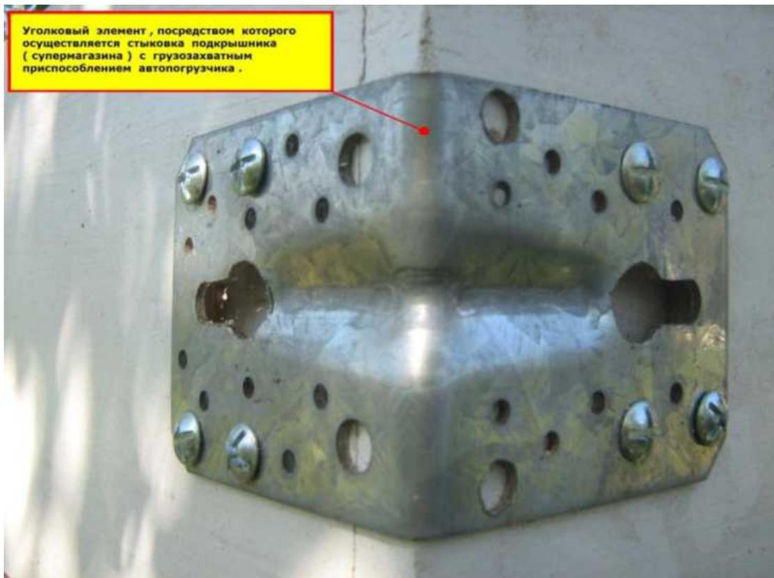
*Fig.8. Element of dock of superstore “Sb – 2008” with the forklift lifting devices.*
