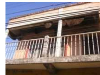
Residential building, Saradanagar
