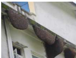
Residential building, Deughat
